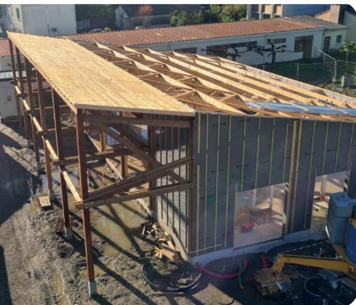
Photo : Fourcade Constructions
